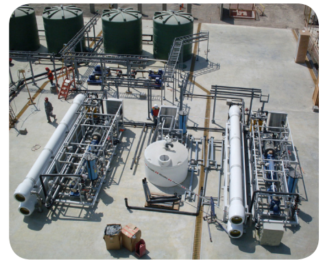
RO Installation at Michilla
