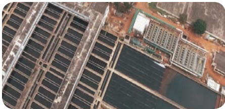
Alto da Boa Vista Drinking Water Treatment Plant, São Paulo, Brazil
